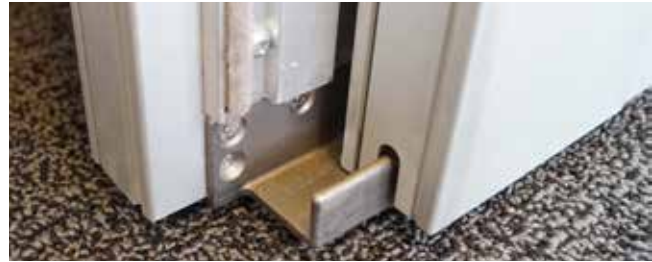
Collection system fixed to doors (not visible when installation is complete).
